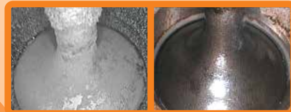
BEFORE: Intake valve with heavy buildup of carbon deposits
